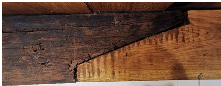
Figure 5. Longitudinal joining of planks
